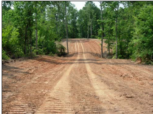
Newly Constructed Road to Parcel B
